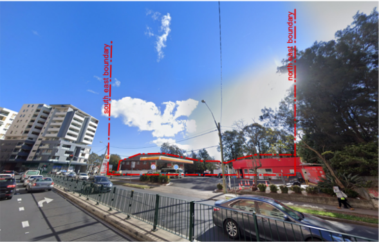
1. view looking west from raw square
