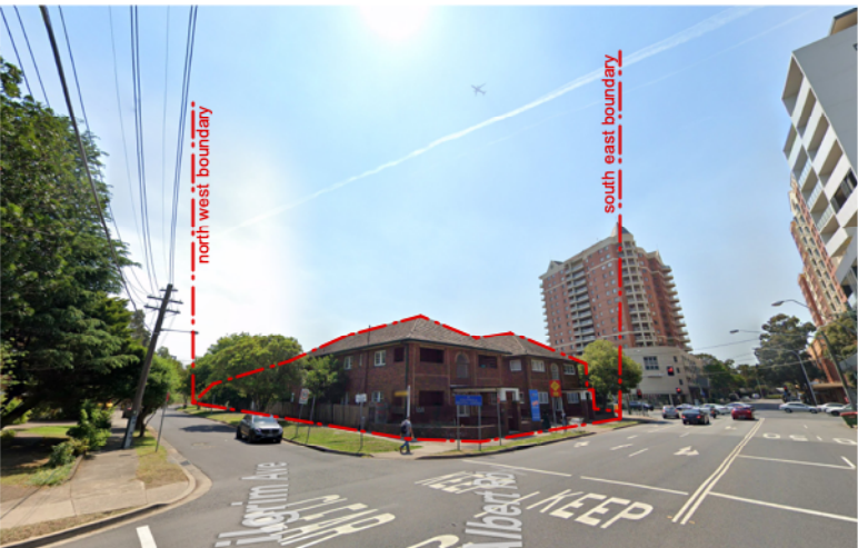
3. view looking north-east from corner of pilgrim ave and albert road
