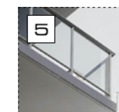
balustrades clear glass within powdercoated aluminium frame Colorbond 'surfmist'
